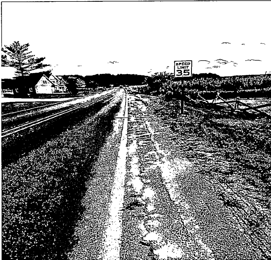
Figure 4 - Longbridge Road looking east toward Pentwater Lake and Marsh showing agricultural lime spread to neutralize the wastewater.
